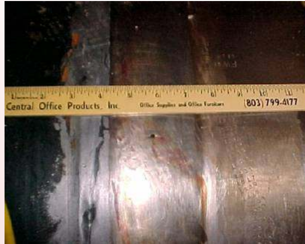
RCS Hot Leg Leaks
