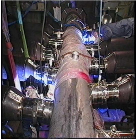
*Phenix : repair of the SG sodium inlet header*
