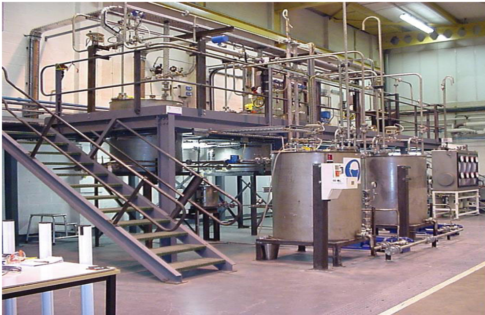
Waste Processing and Handling Mockup (COVE, United Kingdom).
