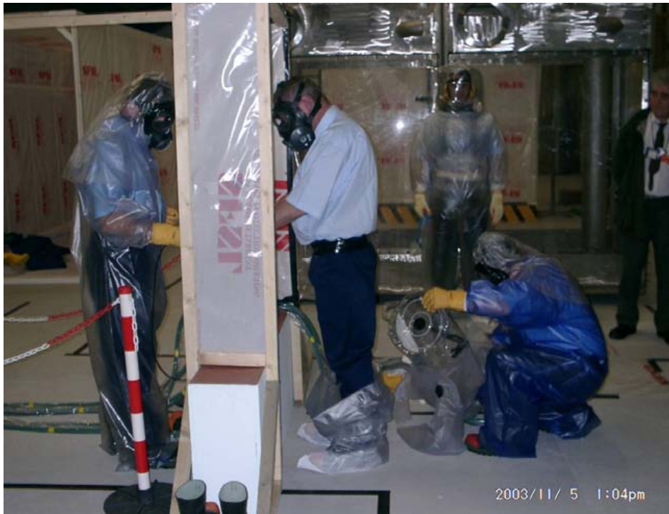
Simple mockup of an entry barrier used to simulate restricted access and develop dressing/undressing procedures (Dounreay, United Kingdom).
