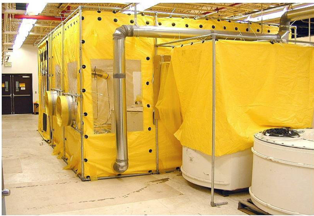
Size reduction tent showing exhaust ducting and waste receptacles.
