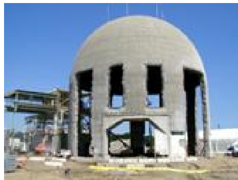
Containment Building Shell, Yankee Reactor Decommissioning Project Maine, USA.
