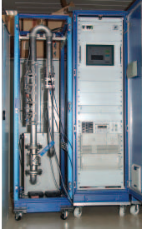
FIG.. 36. Advanced Thermo-hydraulic Power Monitoring.
