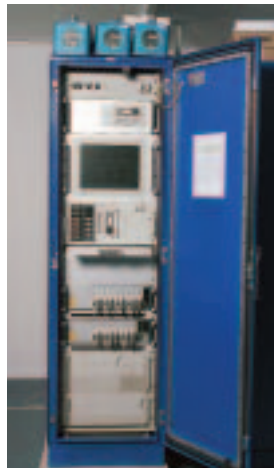
FIG. 27. DMOS: Digital Multi-Camera Optical Surveillance.
