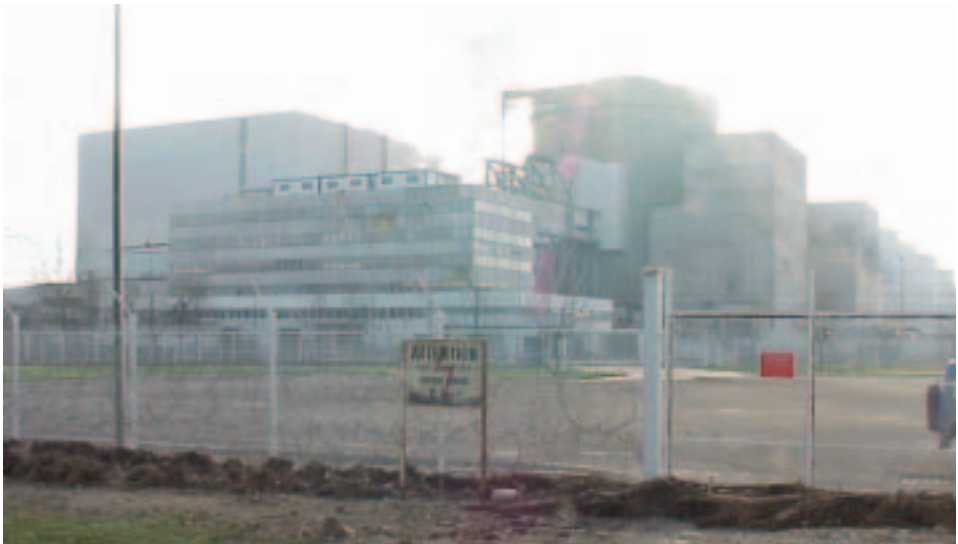
Debris accumulation outside the chain-link fence indicates water level above the site platform (source: IRSN, France).
