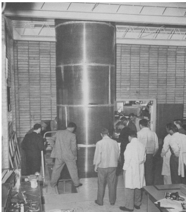
FIG. 4. TRIGA Mark I reactor tank being installed (courtesy of General Atomics).
