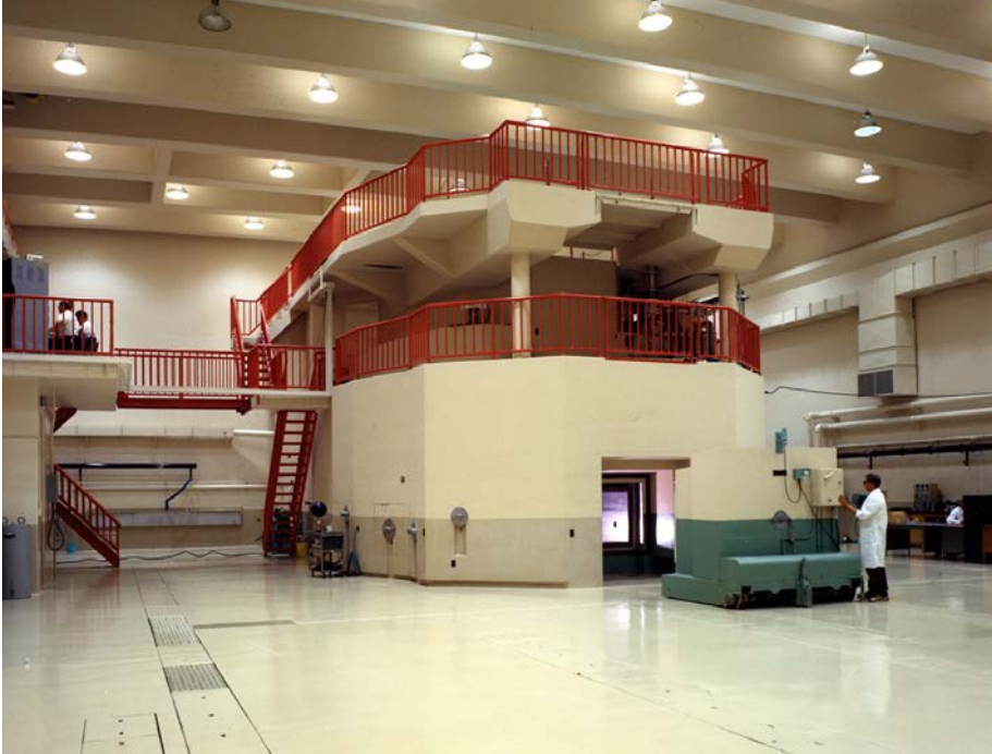
FIG. 19. TRIGA Mark III shield structure and exposure facility at University of California, Berkeley, United States of America (courtesy of General Atomics).
