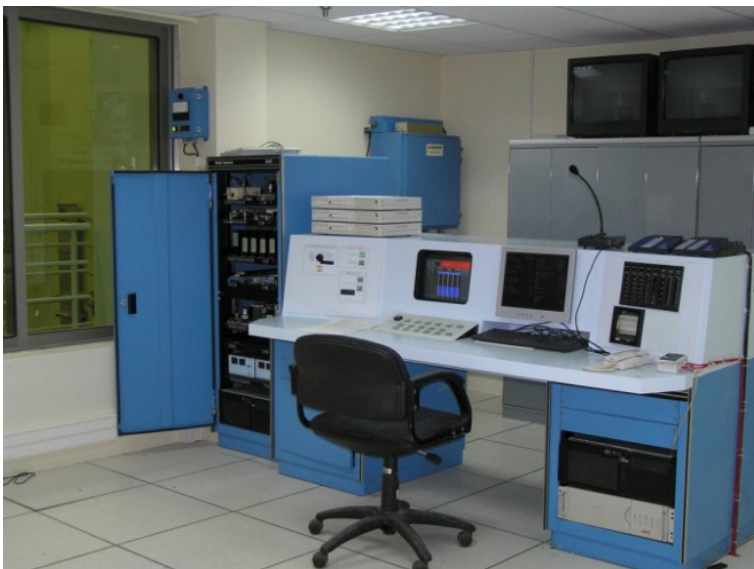
FIG. 40. With the evolution of desktop computers, PC based I&C systems were introduced and various designs continue to be in use today (courtesy of General Atomics and CNESTEN, Morocco).
