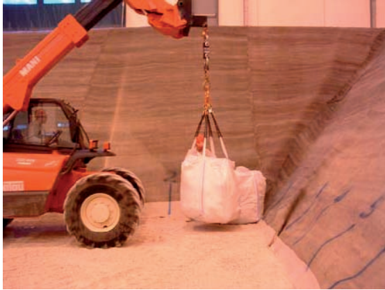
FIG. 6. Morvilliers VLLW site disposal of the first packages.
