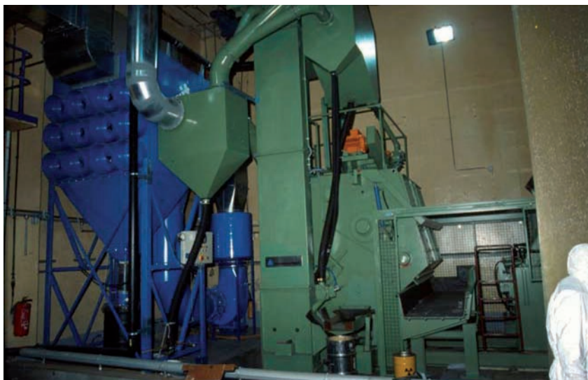
FIG. I-2.2. Operational view of the abrasive blasting installation.
