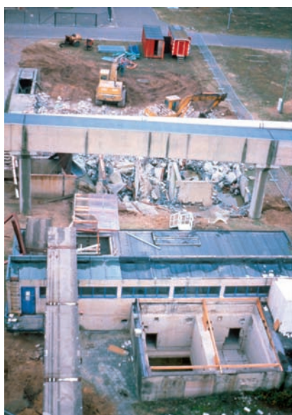
FIG. I-1.2. Demolition of buildings 6A/6B.
