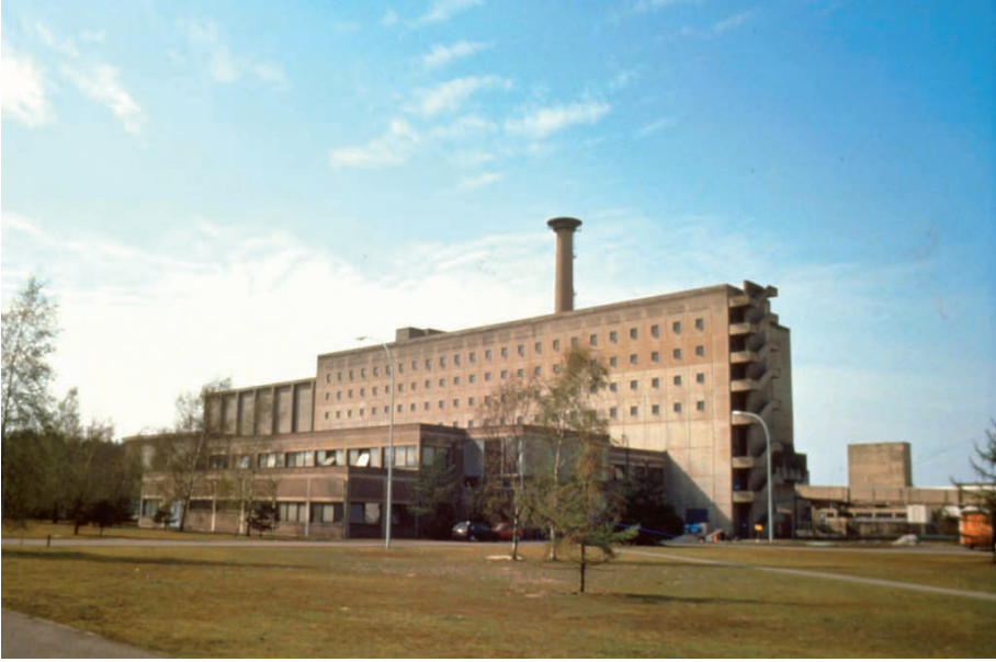
FIG. I-1.1. Main process building of the former Eurochemic reprocessing plant.
