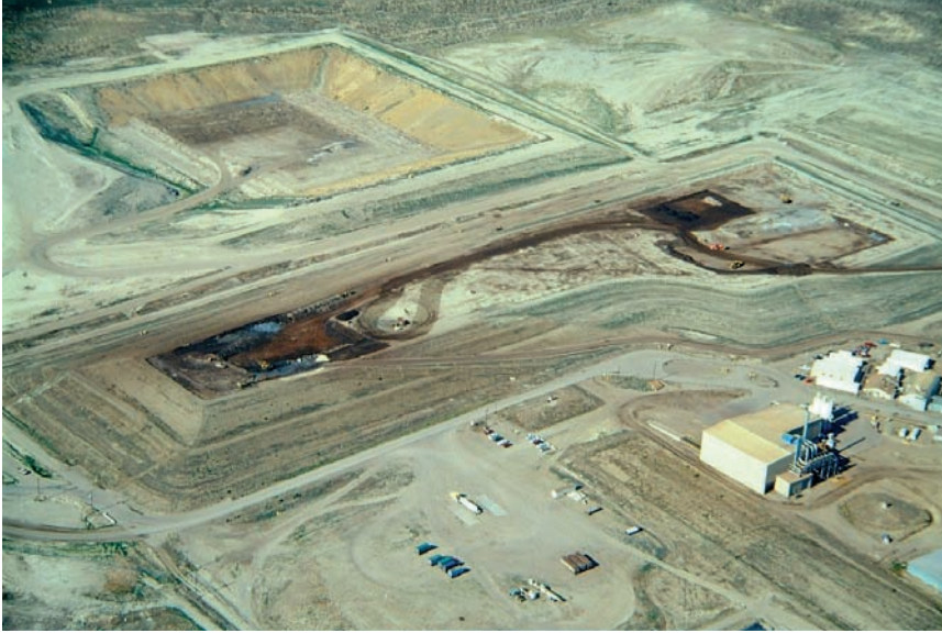
FIG. I-8.2. Newly constructed lined disposal trench.
