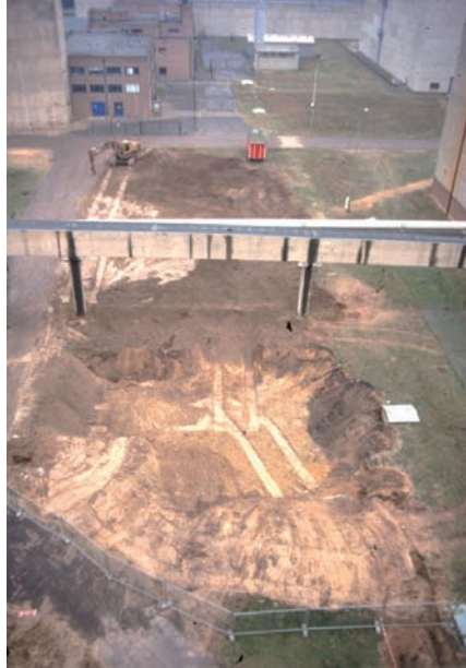
FIG. I-1.3. Green field conditions after demolition of buildings 6A/6B.
