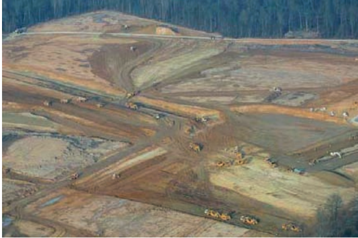
FIG. I-4.4. Earthworks at the construction site.
