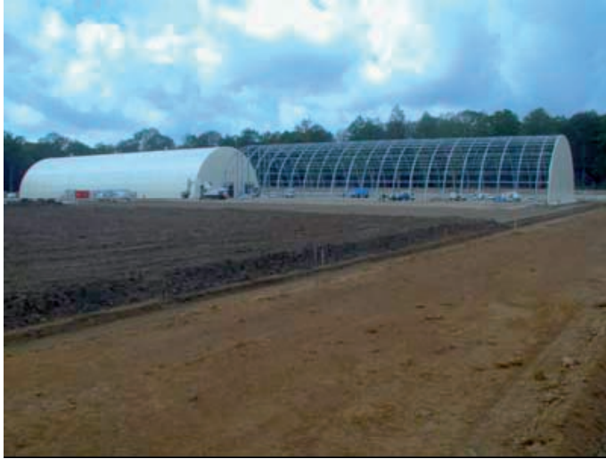
Fig. I-4.5. Construction of the cavities.
