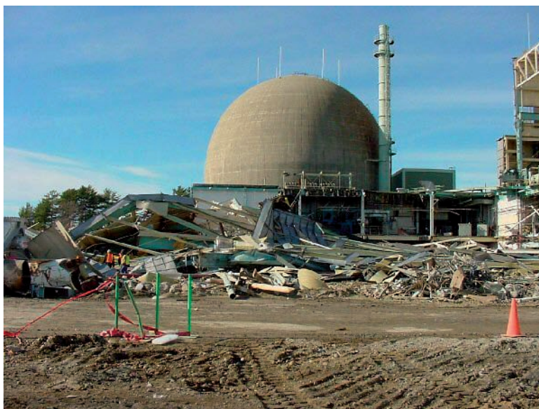
FIG. 2. Maine Yankee nuclear power plant during dismantling.
