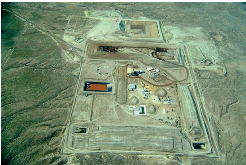
FIG. I-8.1. General view of the Grand View facility.
