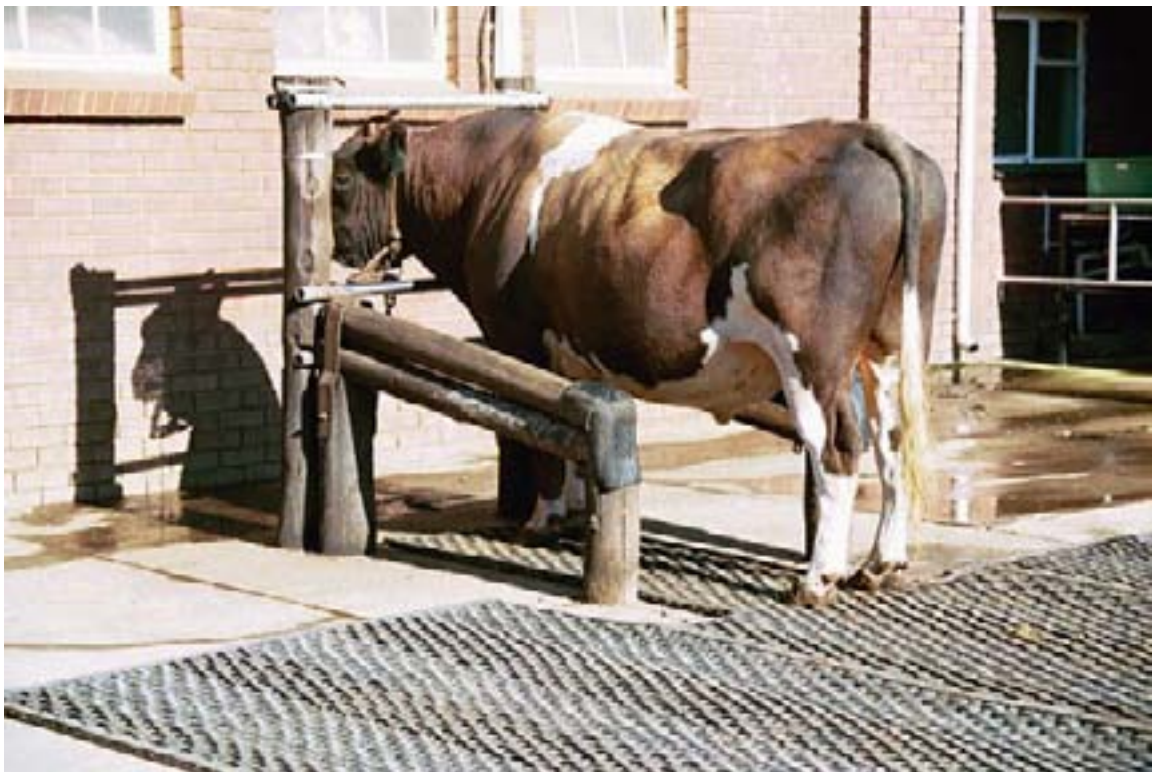
Fig. 3. Strong timber construction of stanchion for teaser bull restraint in South Africa. Note the non-slip floor.
