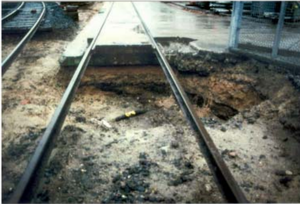
FIG. 13. View after remediation measures at HDR.
