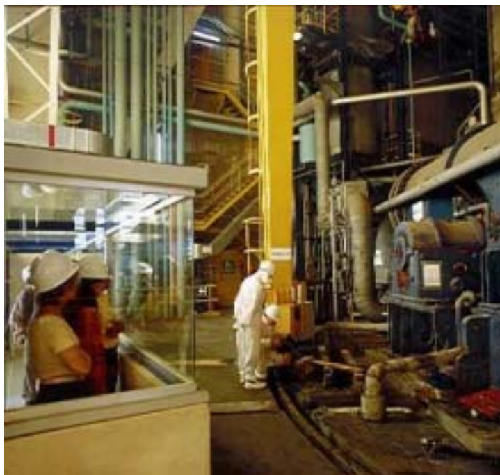
FIG. 6. Vandellos reactor building, “Visiting Point”.
