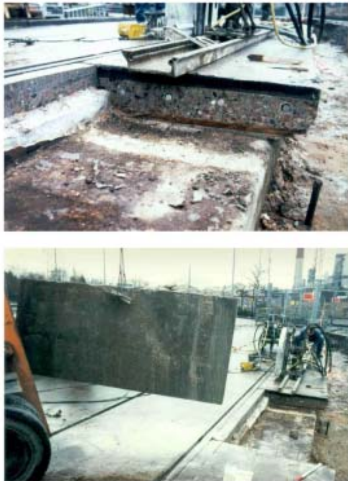
FIG. 12. Segmentation of HDR road to remove contamination.
