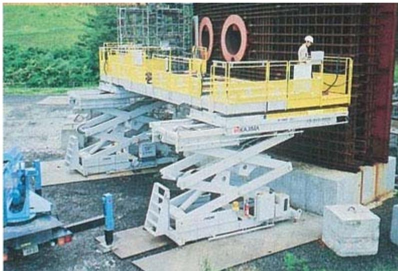
*Fig. 5.19. Automatic elevating scaffolding & horizontal rebar feeding machine (Kashiwazaki-Kariwa).*
