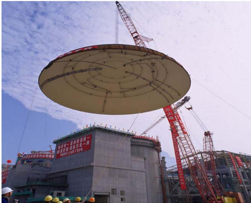
*Fig. 5.15. Lifting of dome module (Lingao).*
