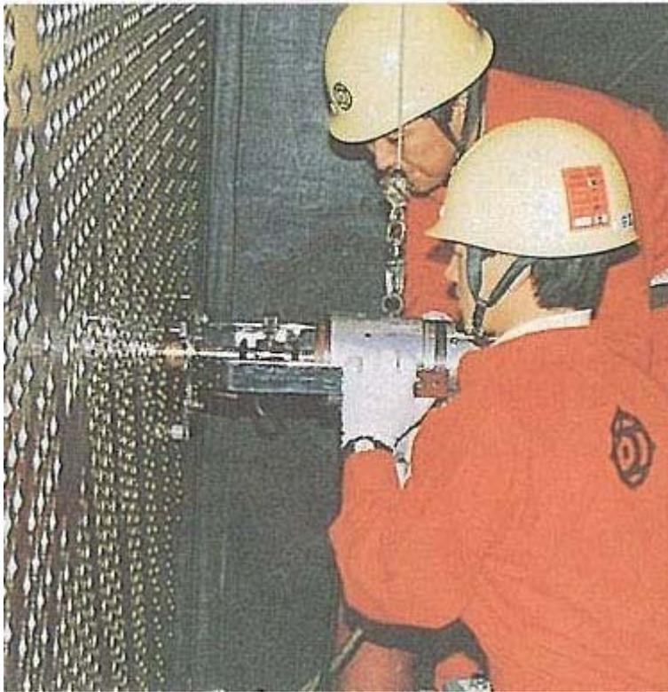
*Fig. 5.18. Automatic welding of condenser tubes (Kashiwazaki-Kariwa).*
