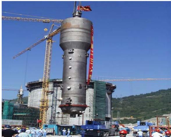
*Fig. 5.5. Steam generator installation (Qinshan).*
