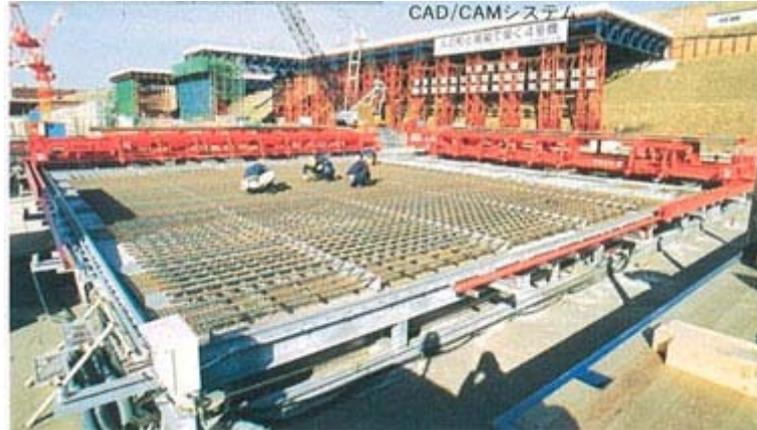
Fig. 5.20. Automatic rebar assembly machine (Kashiwazaki-Kariwa).
