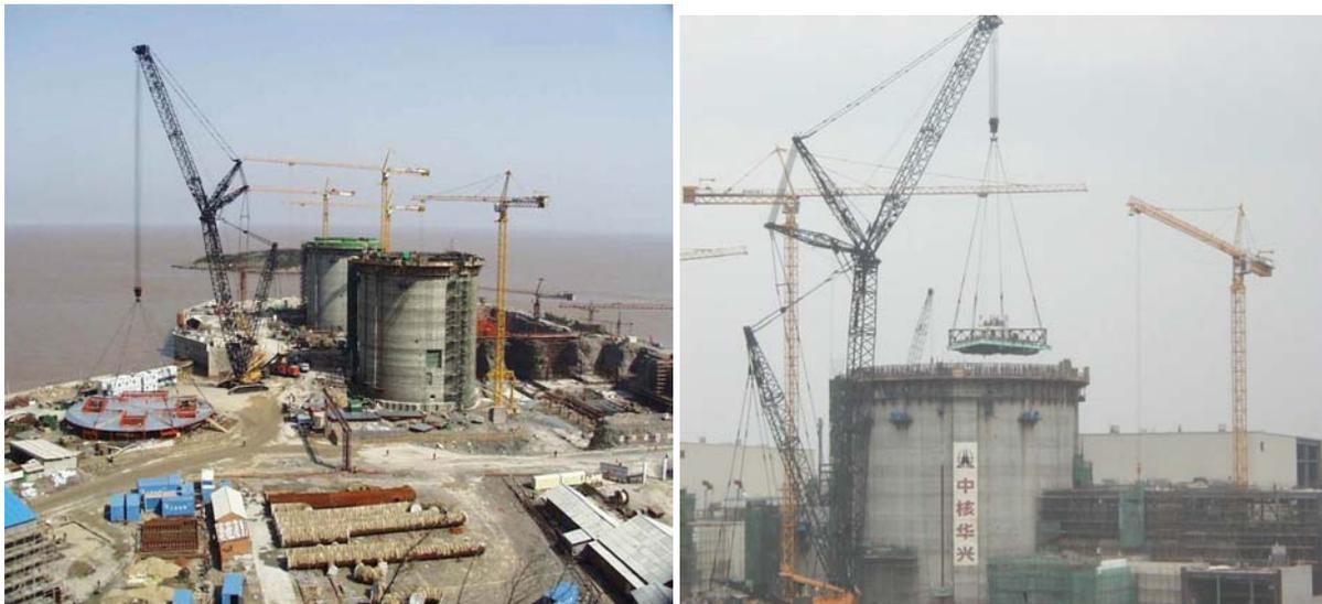
*Figs. 5.3. & 5.4. VHL crane lifting the temporary roof and dousing module (Qinshan).*
