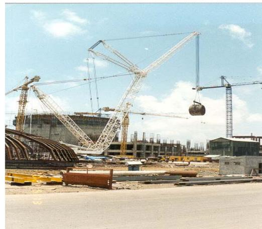
*Figs. 5.6. & 5.7. End shield and calandria installation (Tarapur).*
