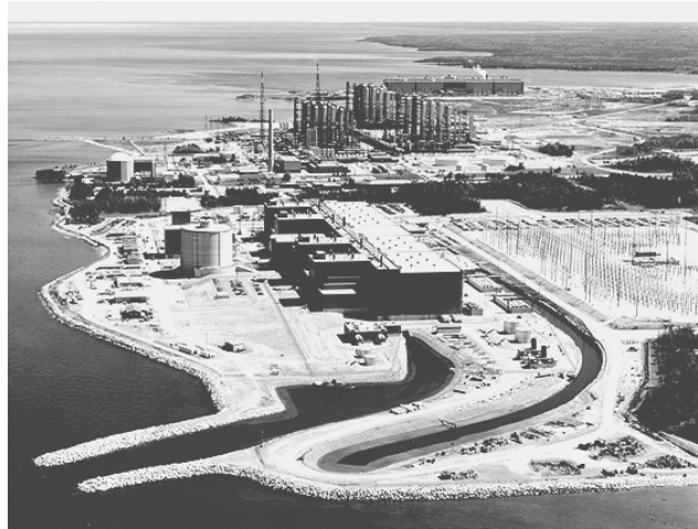
Figure 3. Bruce Nuclear Power Development ( 8 \times 850\text{MW}(e) CANDU units, heavy water production, greenhouse complex using nuclear steam).
