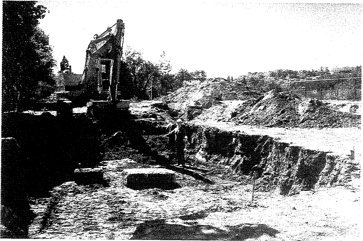
FIG. II-2. Supervised excavation of contaminated soil (Carolyn Street Park), Port Hope, Ontario, Canada.
