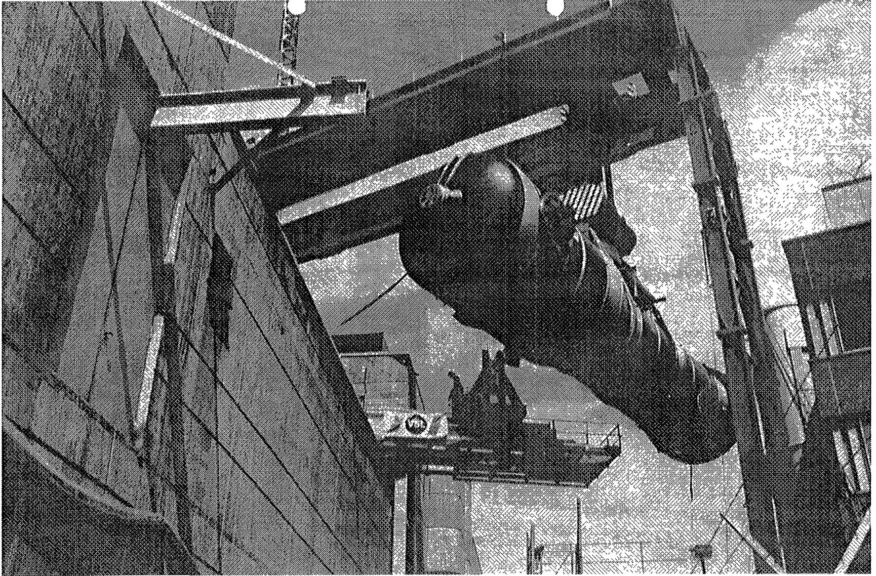
Fig. 8 Exchange of Steam-generators Beznau-1 (1993)
