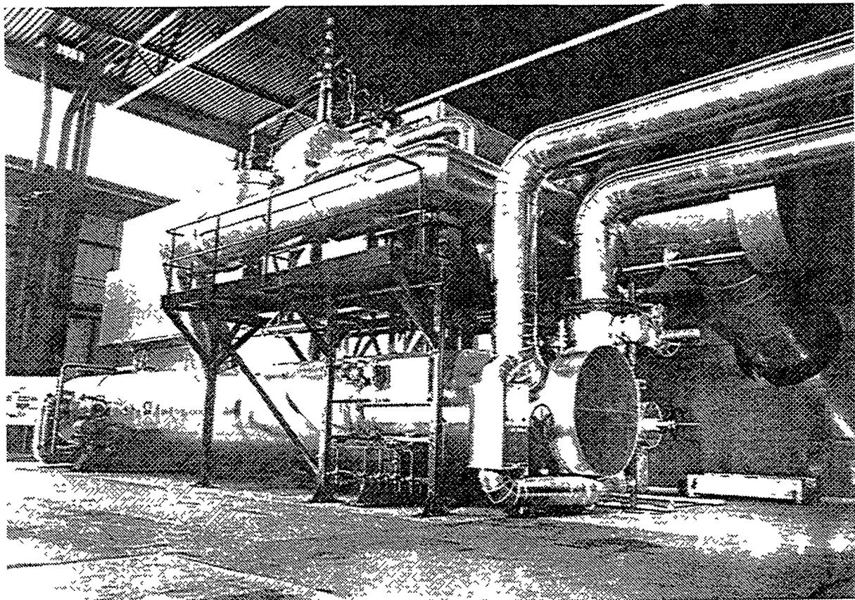
Fig. 3 Large Heat Exchanger of the Beznau Nuclear Plant
