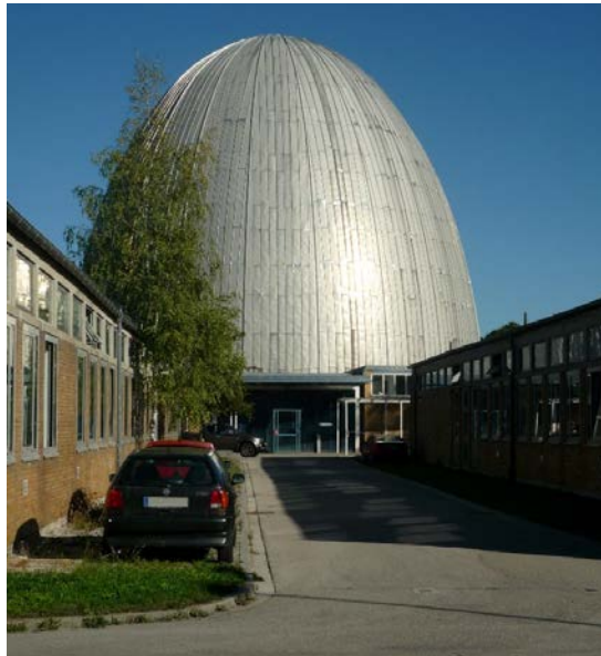
FIG. IV-2. Reactor hall (centre) and low-rise laboratories (left and right) (courtesy of U. Lichnovsky, FRM II, Germany).
