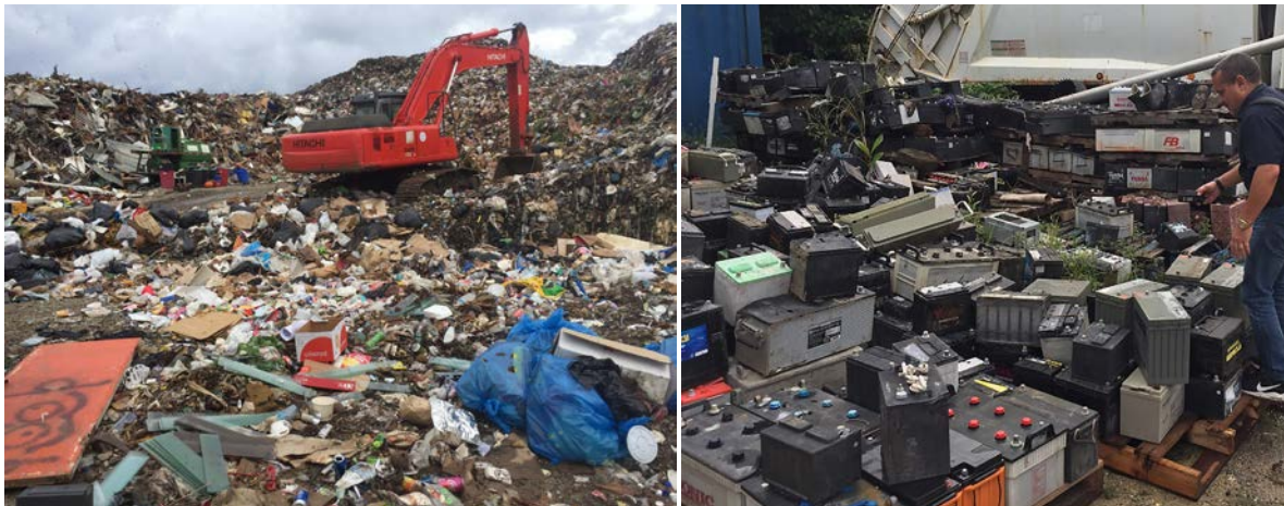
FIG. 9. A landfill where waste is not covered at the end of each day's operation (left) and waste pickers often scavenge for still-usable materials (right).
