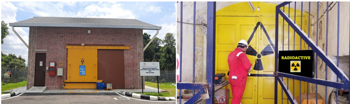
FIG. 26. Examples of entrance to the DSRS storage facilities marked with a trefoil symbol of ionizing radiation and the word ‘radioactive’.
