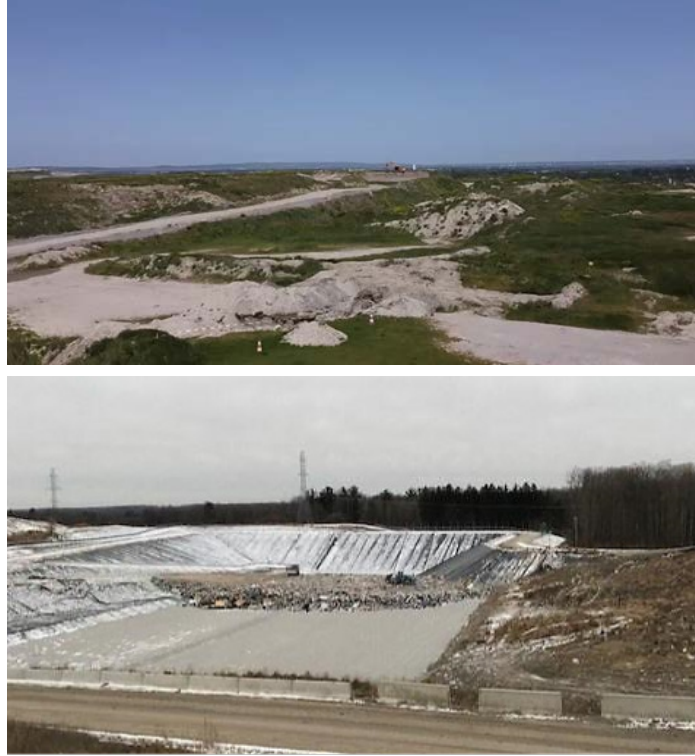
FIG. 8. Example of a well managed landfill where daily waste emplacements are covered.
