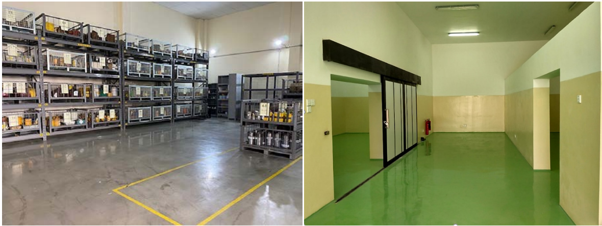
FIG. 25. Example of DSRS storage facilities with proper loading capacity floor and smooth, non-porous surface.
