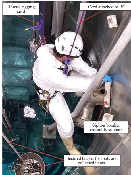
FIG. II-11. Intervention to solve a seizing effect problem.
