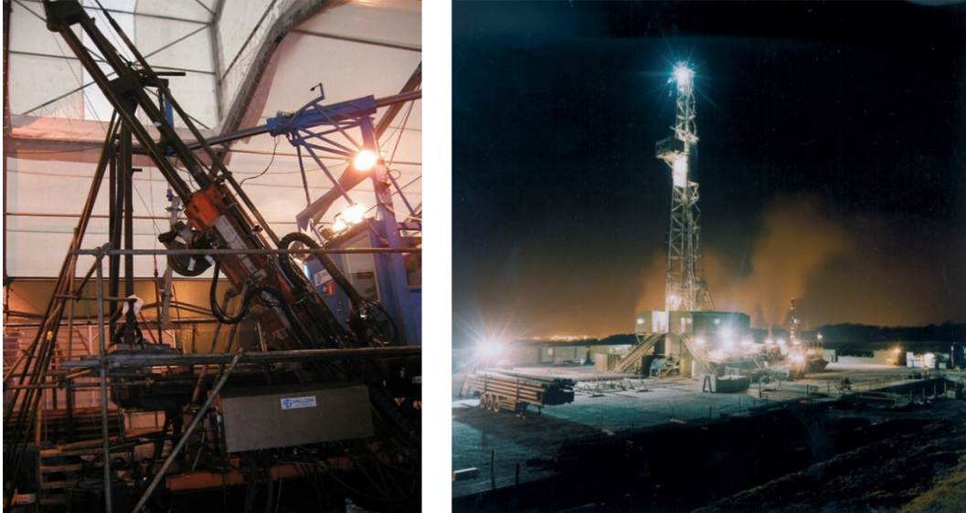
FIG. 28. Drilling rigs used during (a) the Forsmark site investigations in Sweden, and (b) the Sellafield site investigations, UK (reproduced courtesy of SKB and NWS).
