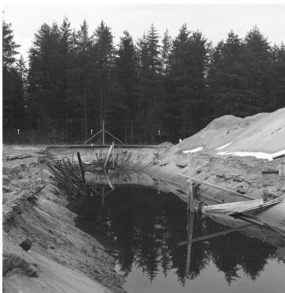
FIG. 15. Liquid waste accumulated in an unlined waste trench at the Chalk River site c. 1953. Photograph courtesy of Atomic Energy of Canada Ltd.
