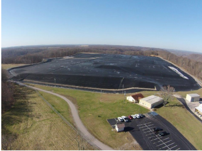
FIG. 10. Aerial photograph of the Maxey Flats site, USA, showing the high density polyethylene geocomposite layer. Photograph courtesy of Commonwealth of Kentucky.
