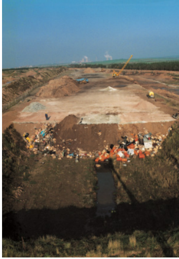
FIG. 1. Historic waste being placed at the Low Level Waste Repository, United Kingdom. Photograph courtesy of Low Level Waste Repository Ltd.
