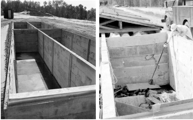
FIG. 33. Single width concrete waste trench constructed at the Chalk River Laboratories site. Left: Empty. Right: with emplaced waste. Photographs courtesy of Atomic Energy of Canada Ltd.
