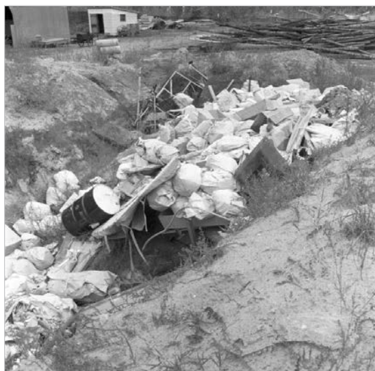
FIG. 32. Typical unlined waste trench with waste dug in the sand at the Chalk River Laboratories site. Photograph courtesy of Atomic Energy of Canada Ltd.
