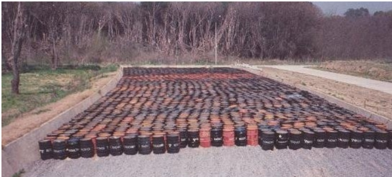
FIG. 2. Drummed historic waste, adjacent to covered trenches containing other drummed historic waste, at the Ezeiza site, Argentina. Photograph courtesy of Centro Atómico Ezeiza.
