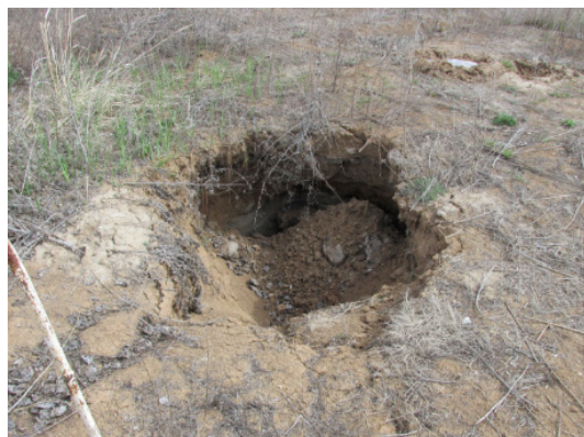
FIG. 13. Void created by the collapse of a trench cover at the ‘3rd Stage of Chornobyl nuclear power plant’ burial site, Ukraine. Photograph courtesy of D. Bugai, Institute of Geological Sciences, Kiev.
