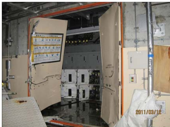
FIG. 32. Damaged door of the heat exchanger buildings. Reproduced courtesy of Tokyo Electric Power Company [64].
