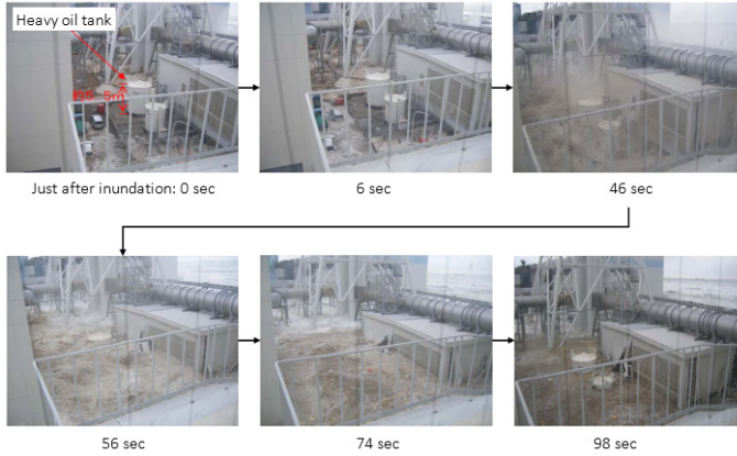
FIG. 20. Inundation near Unit 4 at Point 8 of Fig. 19. Reproduced from Ref. [63] with permission courtesy of Tokyo Electric Power Company.
