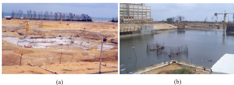
FIG. 12. View of the excavated pit for the PFBR before and after the tsunami. Part (a) is a view of the excavated pit a few months before the tsunami [45]. Part (b) is a view of the excavated pit after the tsunami [46].
