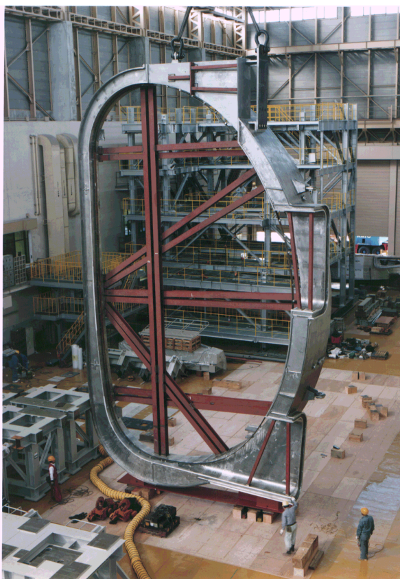
FIG. 1 View of the ITER full-scale vacuum vessel sector A
