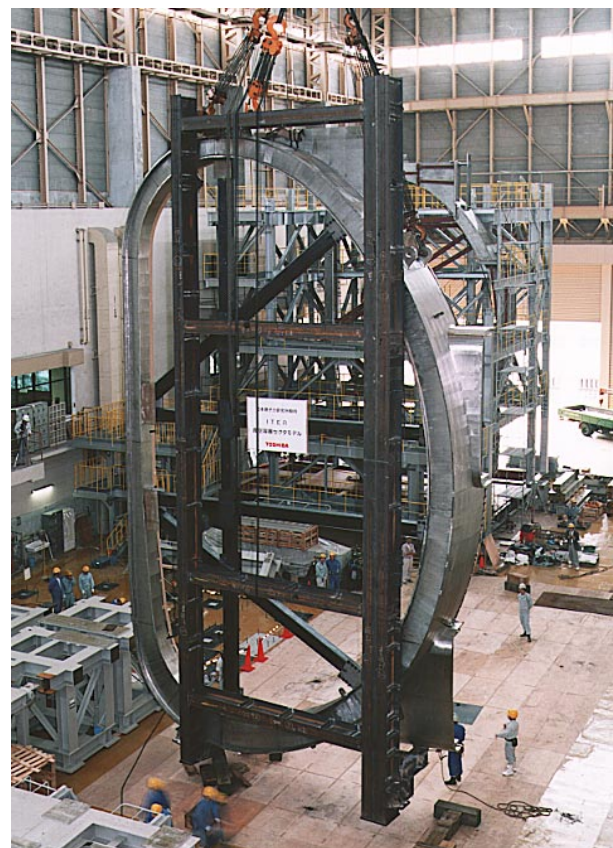
FIG. 2 View of the ITER full-scale vacuum vessel sector B
