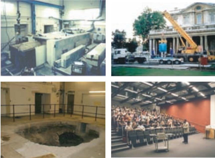
*FIG. 13. Decommissioning of the JASON reactor. Top left: during dismantling operations; top right: removal of spent fuel; bottom left: reactor's pit after dismantling; bottom right: current state, a lecture theatre.*
