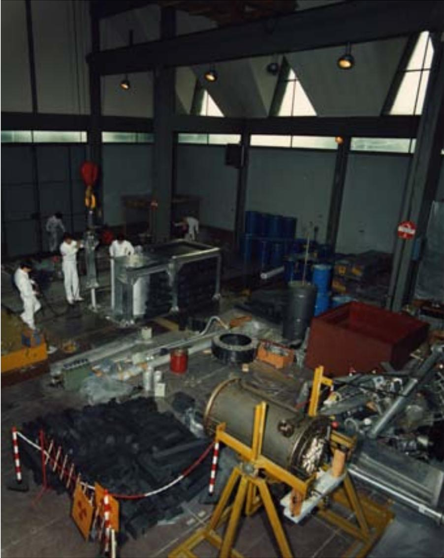
*FIG. 15. RB-2 reactor. Reactor hall floor during dismantling.*
