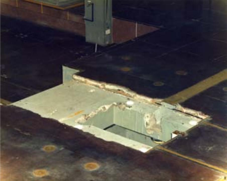
*FIG. 14. RB-2 reactor, Montecuccolino, Italy. Reactor hall floor after removal of the reactor (1986).*
