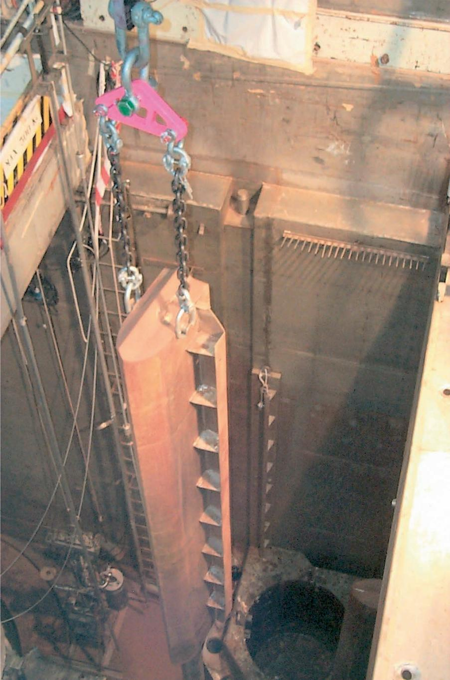
*FIG. A-9. Removal of the last element of the shielding wall.*
