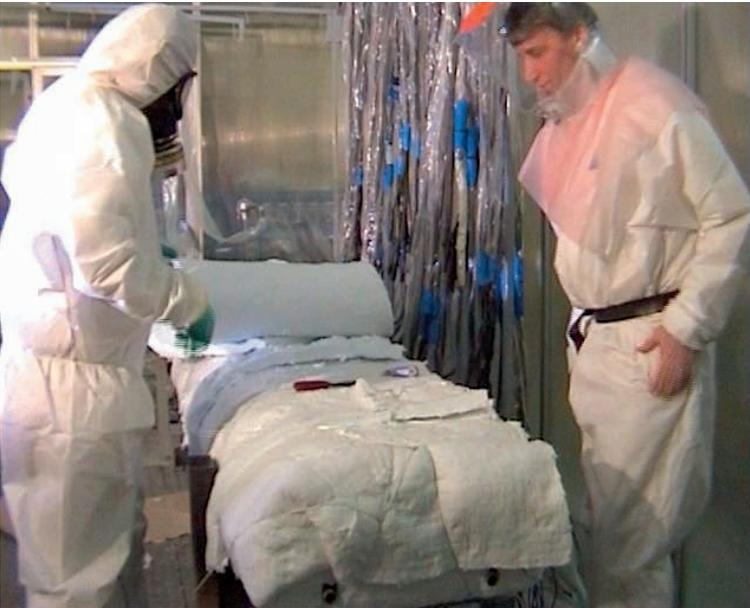
*FIG. A-11. Placement of the insulation material.*
