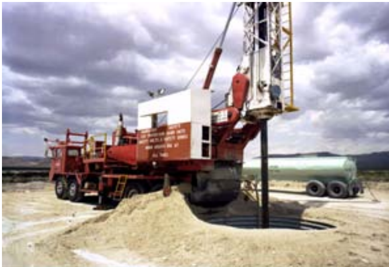
FIG. A-2. Drilling of a Greater Confinement Disposal Facility shaft [A-2].
