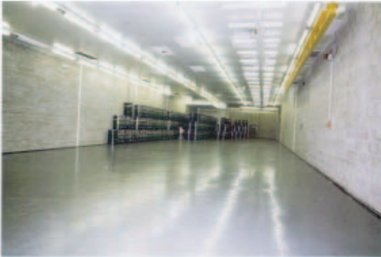
FIG. 26. The PCM drum store, originally the final assembly and pin preparation area of the PFR fuel fabrication plant at Sellafield (after decommissioning).
