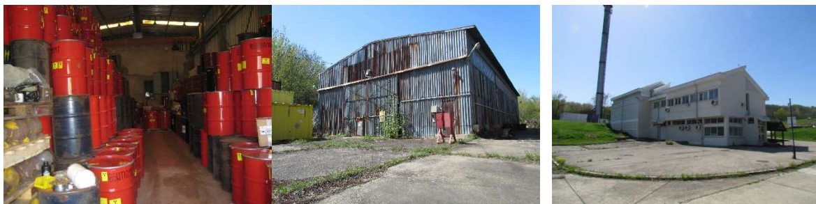
FIG.10. Hangars 1 and 2 and the new processing facility from Vinca site (Photo courtesy of Public Company Nuclear Facilities of Serbia - PC NFS)
