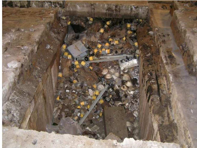
FIG. 3. Example of radioactive waste (in 2006) in RADON facility in Tammiku, Estonia (Photo courtesy of Estonian Waste Management Organization A.L.A.R.A)
