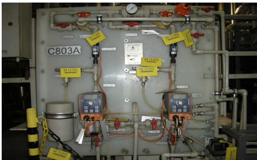
FIG. 68. Automatic dosing system for hydrazine at Bohunice NPP (Courtesy of Slovenské elektrárne, a.s.)
