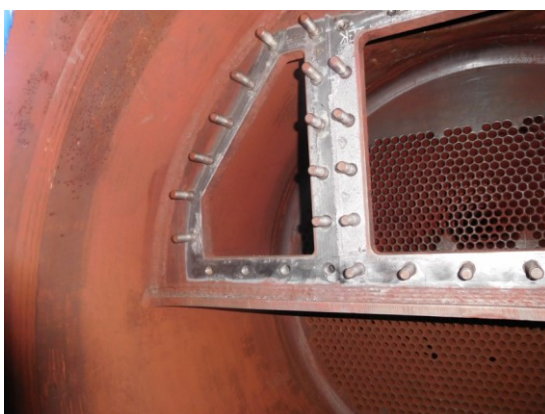
FIG. 43. Visual inspection of a heat exchanger after the application of FFS at Krško NPP, showing a hematite layer without sludge or precipitations (courtesy of NEK).
