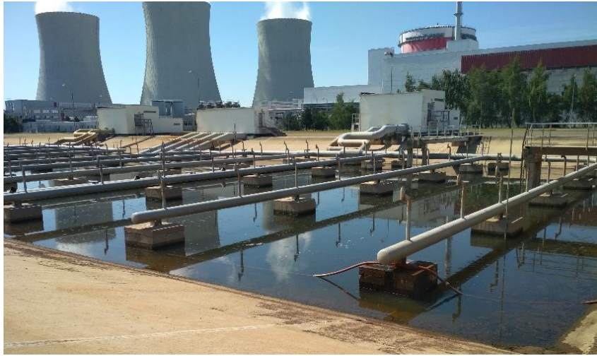
FIG. 59. Spray ponds at Temelín NPP (courtesy of Temelín NPP).
