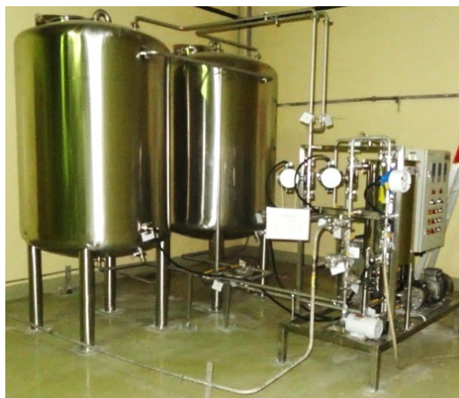
FIG. 11. Qinsan-I filtration system to remove silica in borated water. (courtesy of CNNP).
