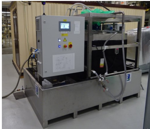
FIG. 39. FFS injection skid at Krško NPP, side view touch control panel (courtesy of NEK).
