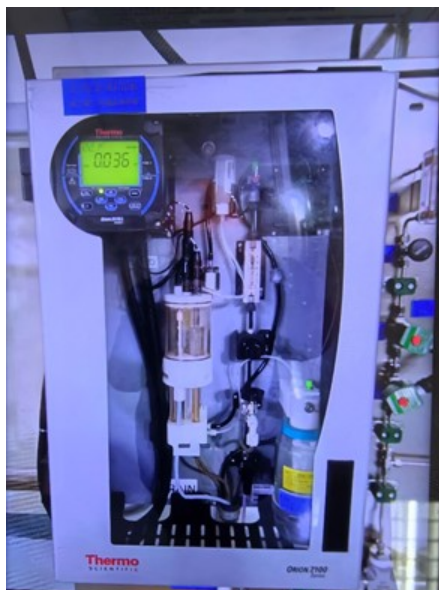
FIG. 67. Online-Na meter used in condenser leakage system at Sanmen NPP (courtesy of CNNP).
