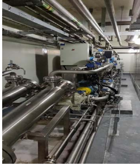
FIG. 9. Picture of the silica removal system installed at Tianwan-I (courtesy of CNNP).
