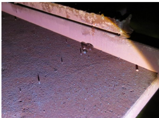
FIG. 41. Visual inspection of condenser, with support structure damaged due to corrosion and hematite layer with minor indications of rust on the upper support structure, after the application of FFS at Krško NPP (courtesy of NEK).
