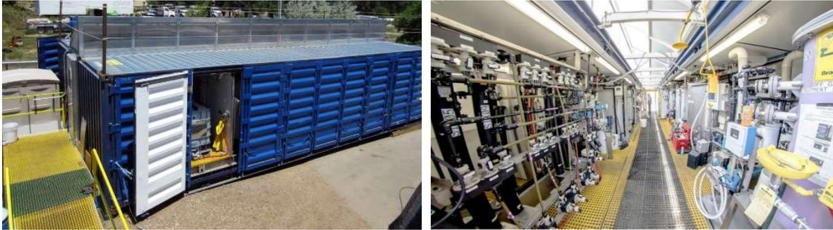
*FIG. 8. PhosEnergy pilot plant that uses an ion exchange process for uranium recovery from phosphoric acid erected in the USA (courtesy of PhosEnergy).*
