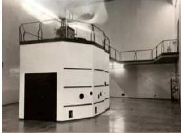
FIG. 3. The L-54M reactor. (Courtesy of POLIMI).
