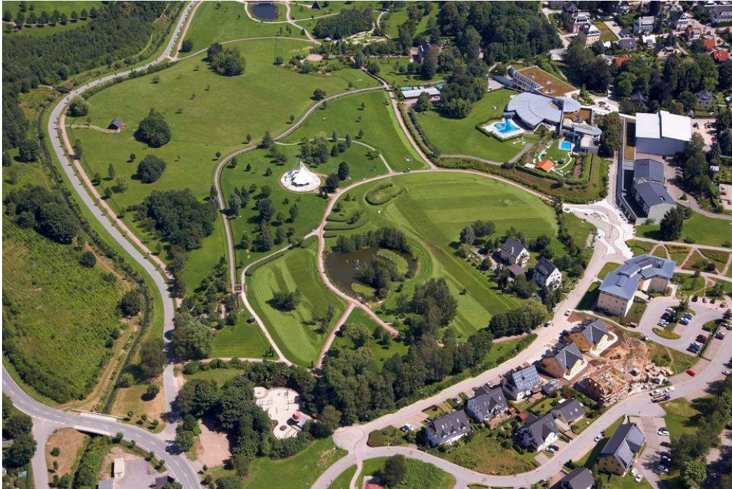
FIG. 7. Aerial view towards the Schlema spa garden, with re-shaped, covered and re-cultivated waste rock piles on the left.
