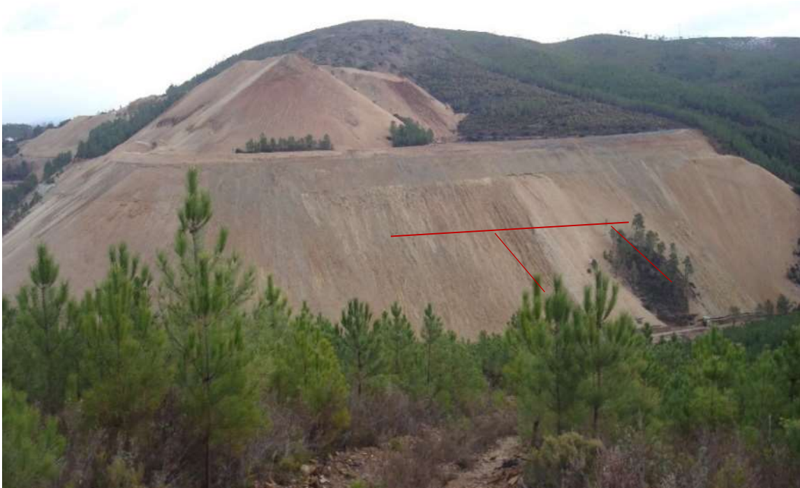
FIG. 14. Most probable area of failure by erosion of the embankment wall and erosion zones below the support wall.
