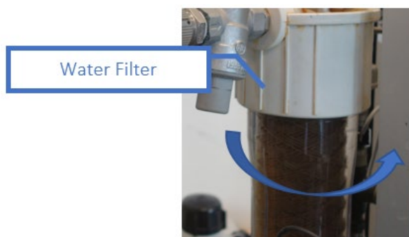
FIG. 13. Water filter casing with an arrow indicating the direction of the turn to close it.
