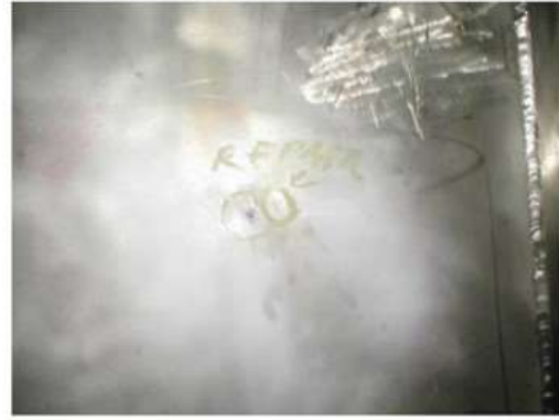
FIG. I-24. Counting of leakage points in transfer channel FIG.I-25. Leak points marking (courtesy of BRIN, Indonesia)
