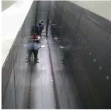
FIG. I-24. Counting of leakage points in transfer channel FIG.I-25. Leak points marking (courtesy of BRIN, Indonesia)
