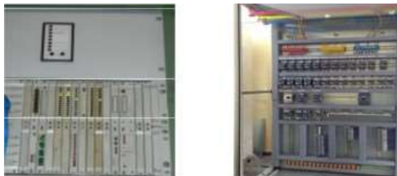
FIG. I-21. (a) Card based controller I/O (Old) (b) MCCP panel (courtesy of NFC, India)
