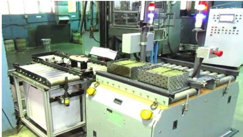
FIG. II-10. Automated Boat Transfer using AGV (courtesy of NFC, India)
