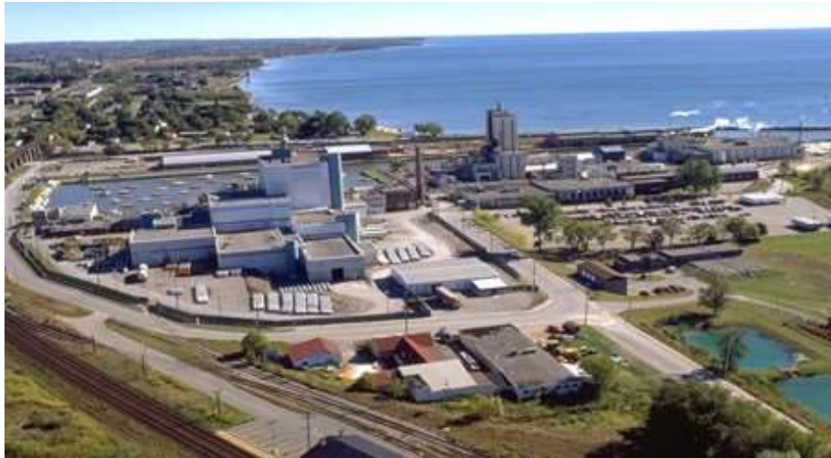
FIG. I-7. Port Hope conversion facility (courtesy of CNSC, Canada)
