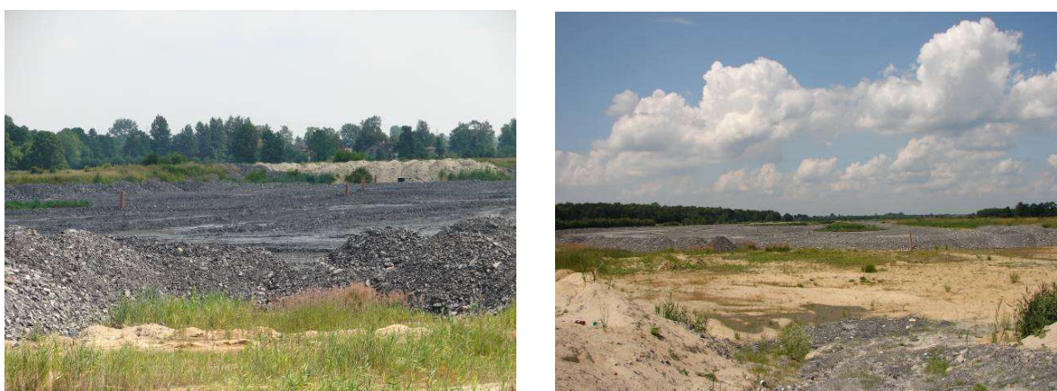
FIG. 82. Photographs of the settling pond area.
