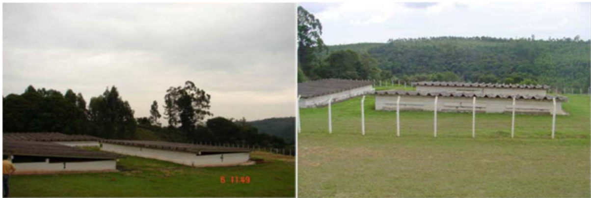
FIG. 24. Silos on the Botuxim site where residues from monazite processing are stored.
