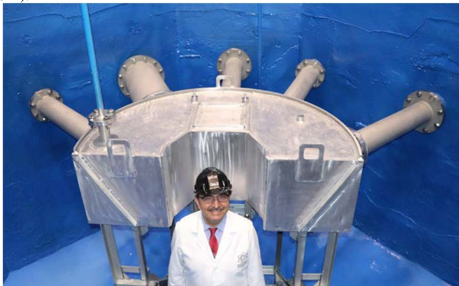
FIG. II-9. Prof. Ünlü inspecting the new D_2O tank and new beam ports before filling the reactor pool and placing the reactor core for proceeding regular operation (courtesy of K. Ünlü, PSBR).
