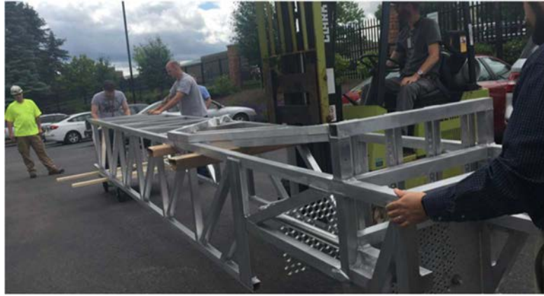
FIG. II-6. Reactor tower with upper and lower grid plates as delivered for installation (courtesy of K. Ünlü, PSBR).
