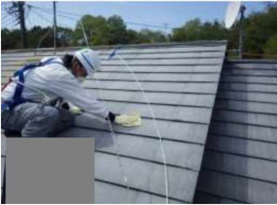
(A). Removal of sediments
