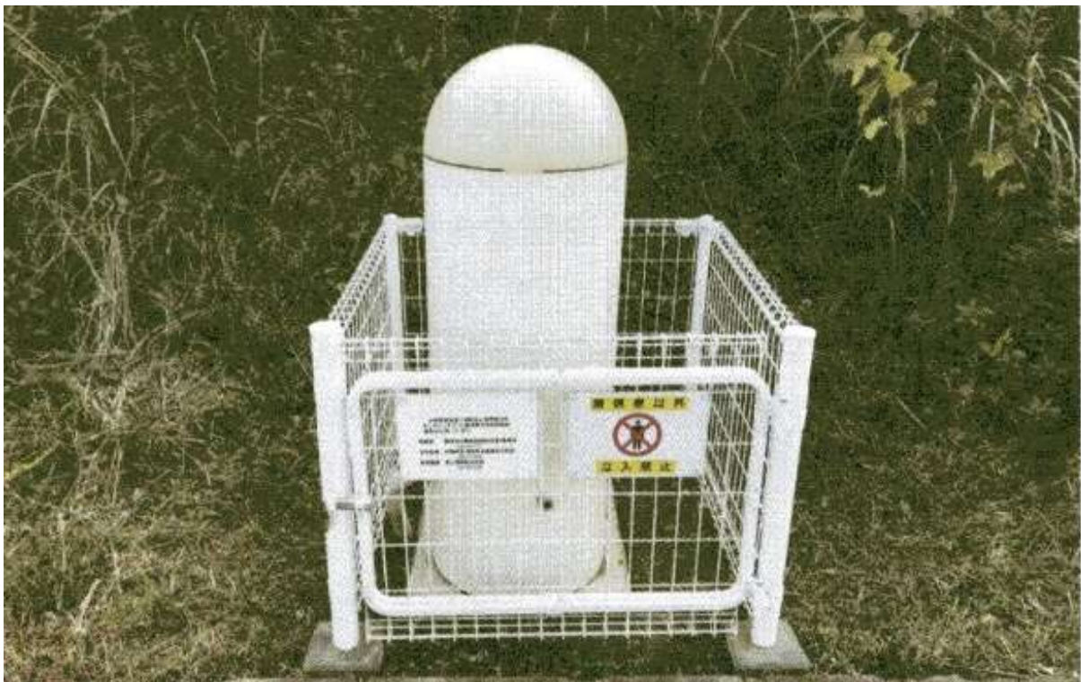
FIG. 27. Dose rate monitoring station for waste transportation (reproduced from [86] with permission).
