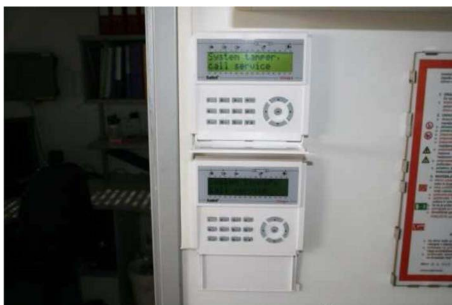
FIG. I-12. Security system commands.
