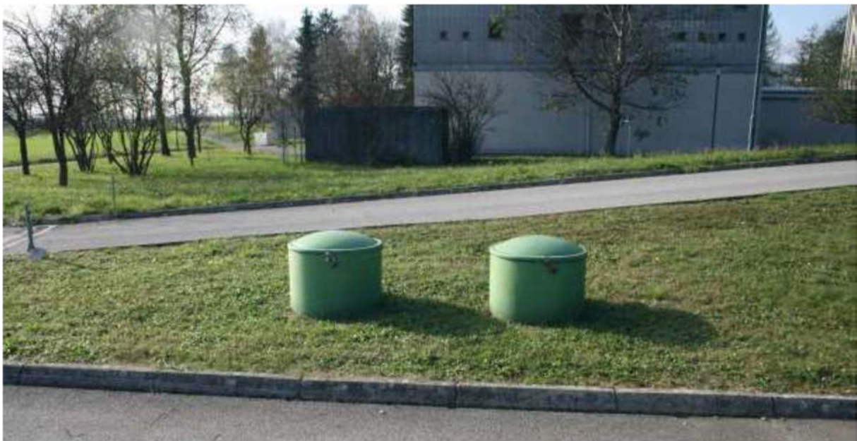
FIG. I-10. System for collection and retention of liquids, outer part.
