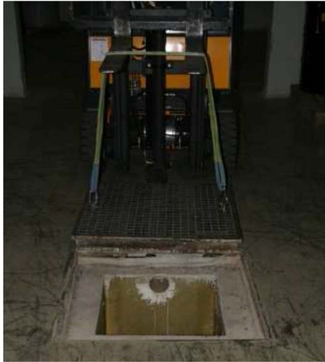
FIG. I-9. System for collection and retention of liquids.
