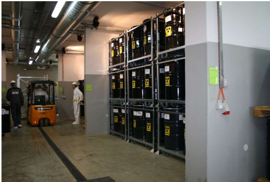
FIG. I-19. Individual storage compartments in the CSF.
