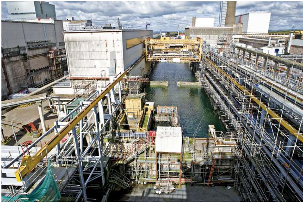
FIG. 5. The First Generation Magnox Storage Pond gantry refurbishment system has successfully completed a key risk reduction enabler for recovery of the pond inventory (courtesy of Sellafield Ltd).
