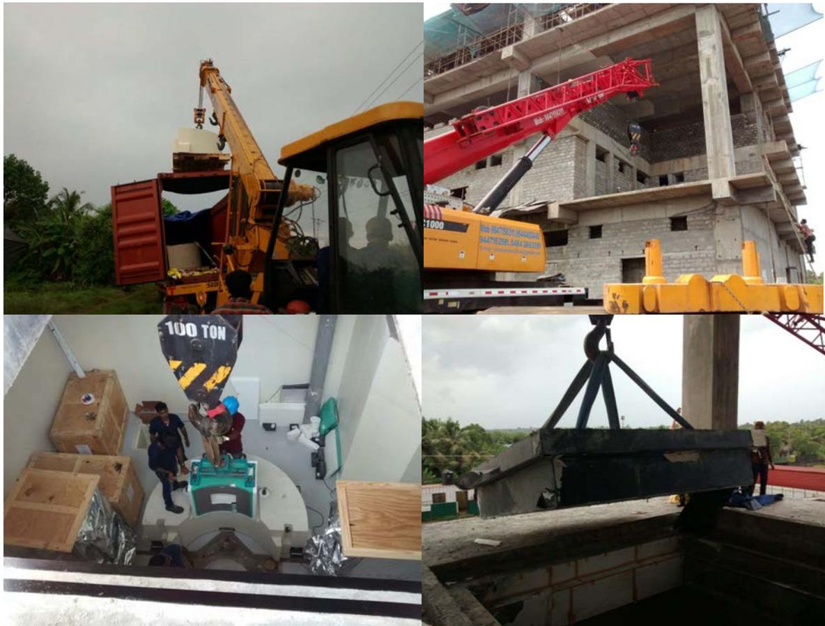
FIG. 94. Example of a cyclotron installation (courtesy of K.N.S. Nair, Molecular Cyclotrons).
