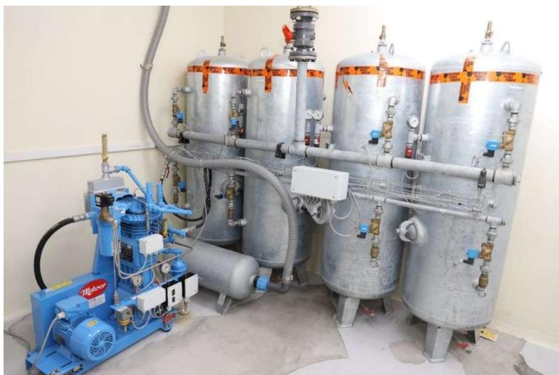
FIG. 103. Delay-decay tanks used in a cyclotron facility (courtesy of K.N.S. Nair Molecular Cyclotrons).
