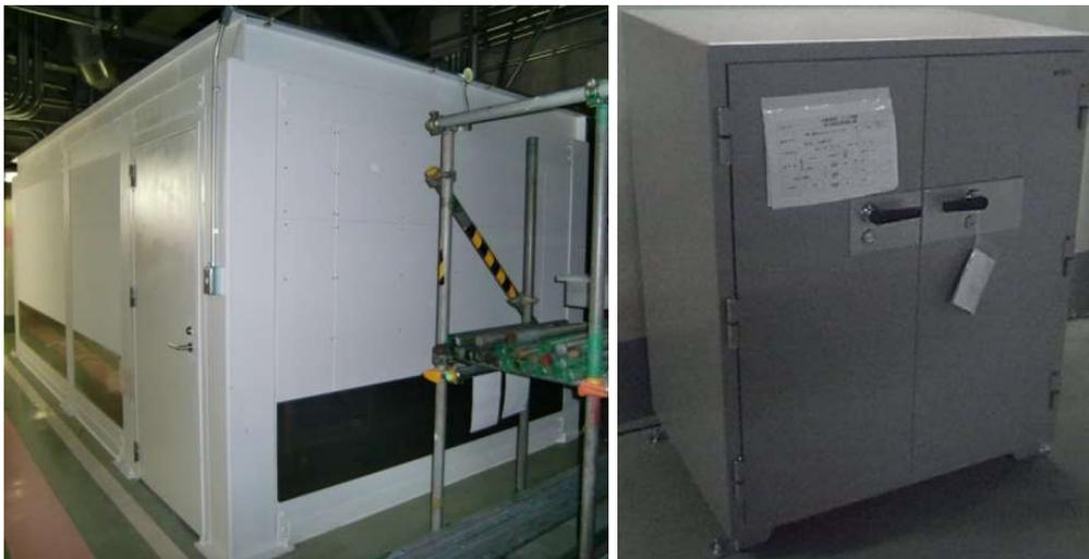
*FIG. 5. Example of fireproof storage facility and fireproof storage container (left to right)*
