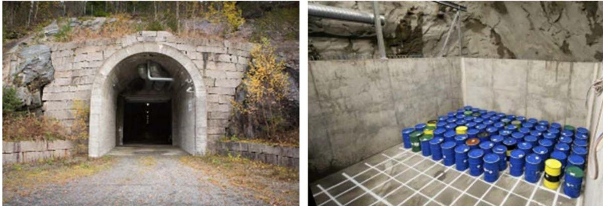
*FIG. 12. Himdalen disposal facility for LLW, Norway (Courtesy of IFE).*
