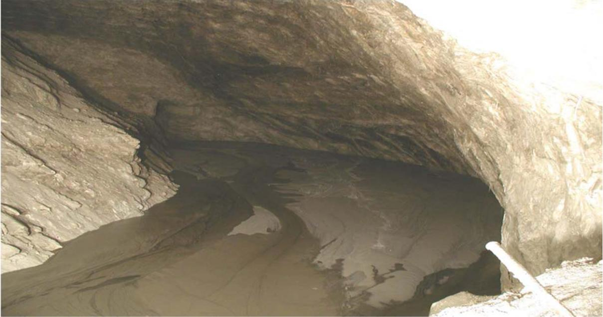
FIG. 30. Picture of backfilling a mine opening as an advanced activity prior to final closure (Courtesy of BGE).
