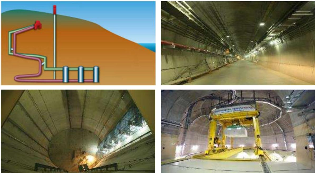
FIG. 15. The Wolsong LILW Disposal Centre (Courtesy of KORAD): schematic view (top left), operating tunnel (top right), disposal silo (bottom left) and waste container emplacement device (bottom right) (from [55]).
