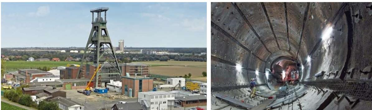
*FIG. 24. The Konrad repository for LLW and ILW: mine shaft (left) and construction of a permanent transport drift (right) (Courtesy of BGE).*
