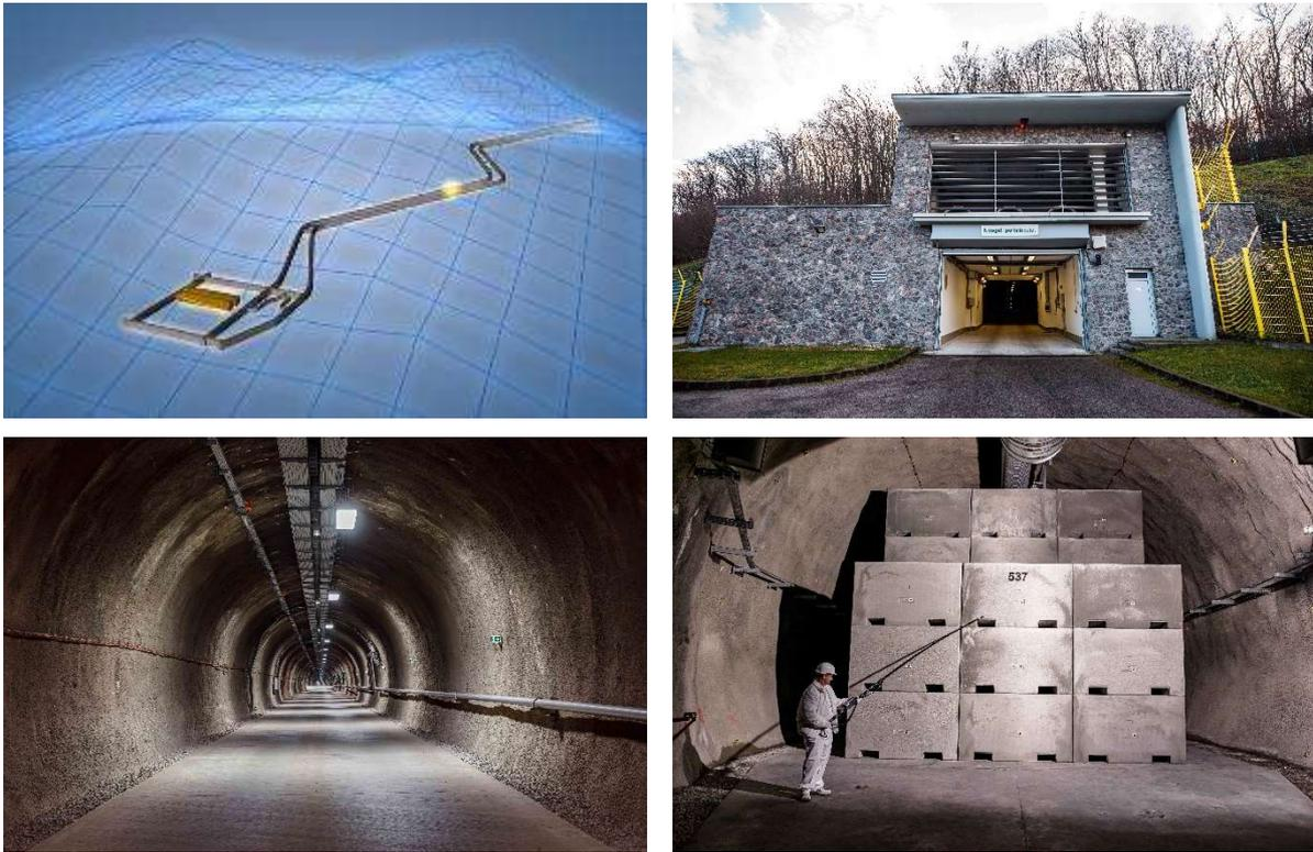
FIG. 13. The National Radioactive Waste Repository in Bataapati (Courtesy of PURAM): schematic view of the facility (top left), facility entrance (top right), access tunnel (bottom left) and emplaced waste containers (bottom right).
