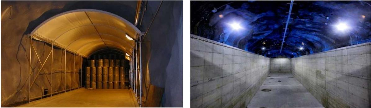
FIG. 20. Hall with LLW waste drums (left) and underground concrete vault for the disposal of ILW containers (right) (Courtesy of FORTUM).
