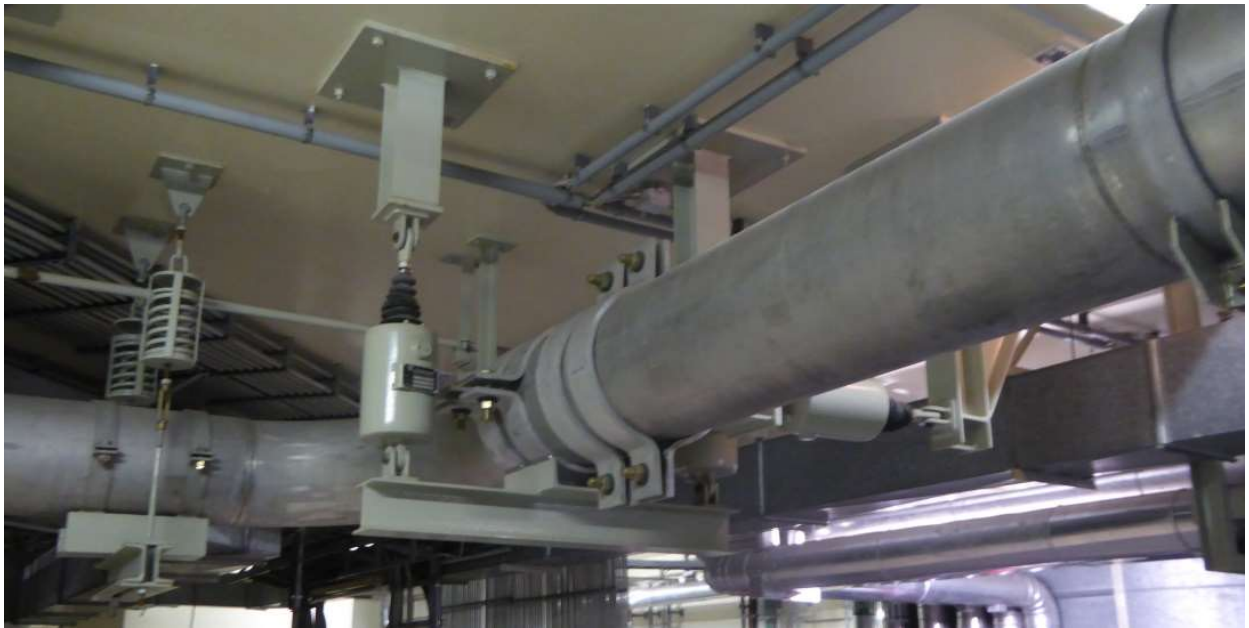
FIG.15. PIPING SUPPORTS
