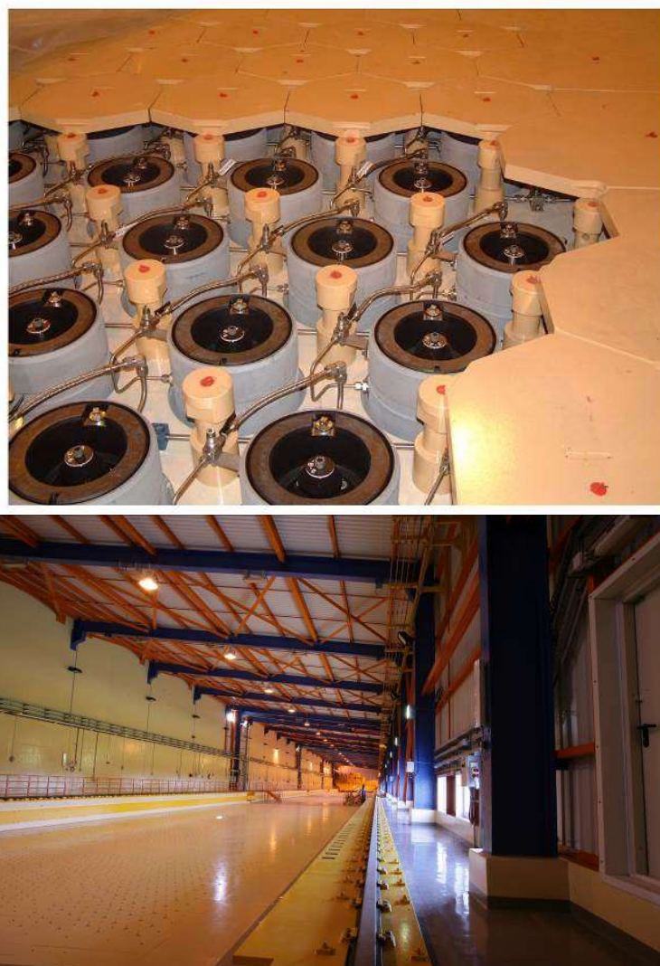
FIG. 7. Paks MVDS, operator PURAM, Hungary. Views of the top of the storage tubes and the charge hall (photographs courtesy of PURAM).
