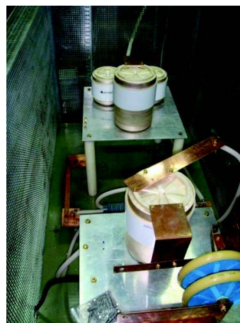
View of RF matching circuit
