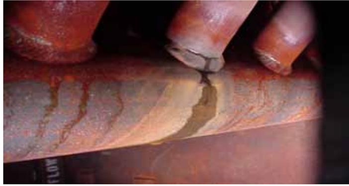
*FIG. 2.4. Leaking tube to header welds provide multiple parallel leak paths.*
