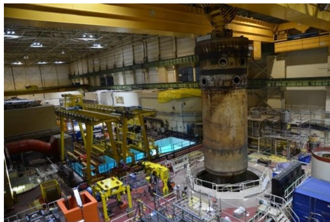
FIG. I-6. Retrieval of the reactor pressure vessel (photo courtesy of JAVYS, a.s.).
