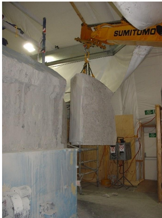
FIG. II-2. Removal of concrete block at Moata reactor, Australia (courtesy of ANSTO).
