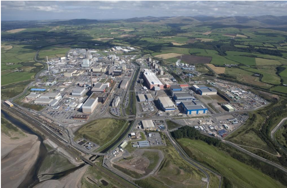
FIG. I-18. Aerial view of the Sellafield site (photo courtesy of Sellafield Ltd).
