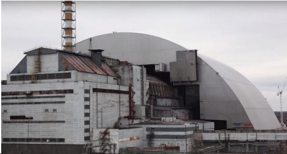
FIG. I-16. Placement of the NSC (photo courtesy of Chernobyl NPP).
