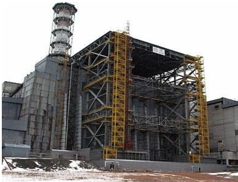
FIG. I-14. View of the Shelter after implementation of stabilization measures (photo courtesy of Chernobyl NPP).
