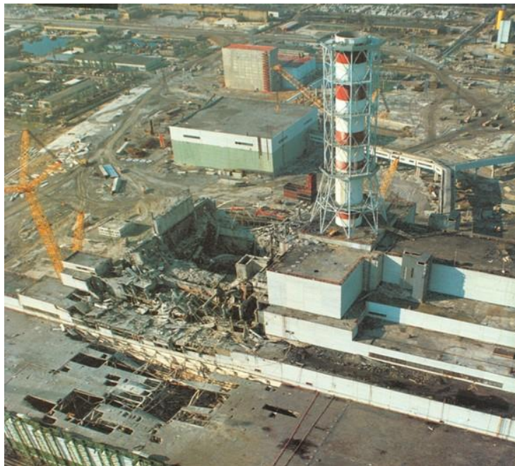
FIG. I-11. Unit 4 of the Chernobyl NPP destroyed as a result of the accident (photo courtesy of Chernobyl NPP).
