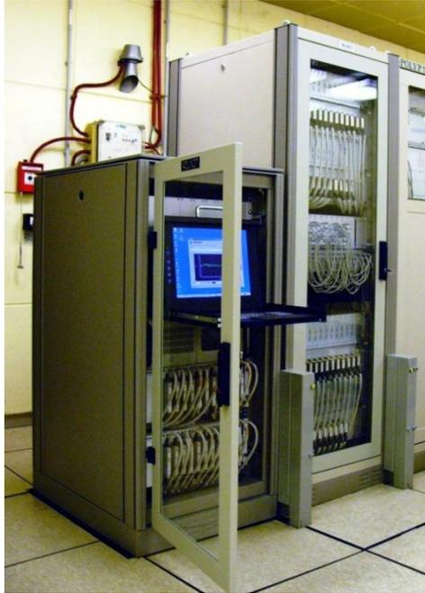
*FIG. 1-4. PAZAR Configuration at Unit 4: system computer and multiplexers are placed in the smaller rack; signal conditioning modules are installed in the larger cabinet.*
