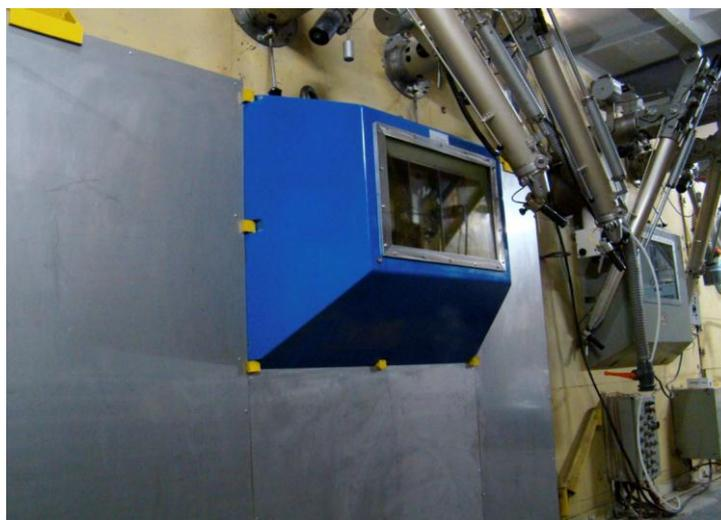
*FIG. 18. New window and additional shielding to radiochemical cell*
