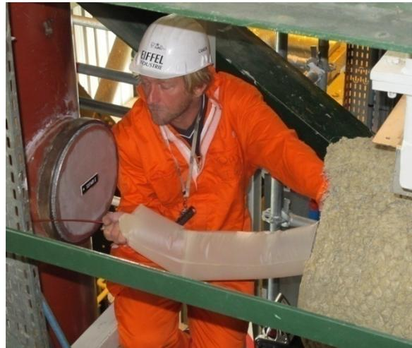
Opening of the sodium circuit with argon and get in of the camera and its support
