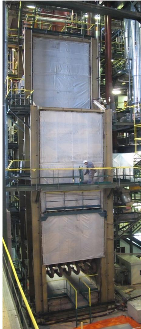
Implementation of curtains for the heating to 50 °C in the steam generator casing
