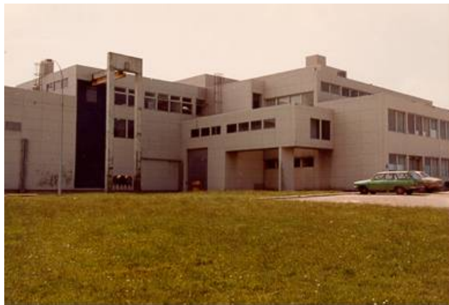
Figure 2: View of workshop AT1
