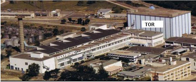
Figure 5: View of the renovated Marcoule pilot workshop.
