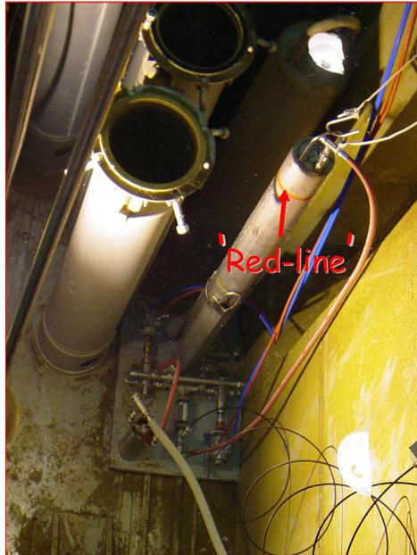
*FIG. 5. RBOF underwater deionizer with empty oversized can halves.*
