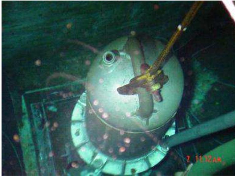
FIG. 3. An oversized aluminium storage can used for damaged-fuel (at -9.14 m) in RBOF.
